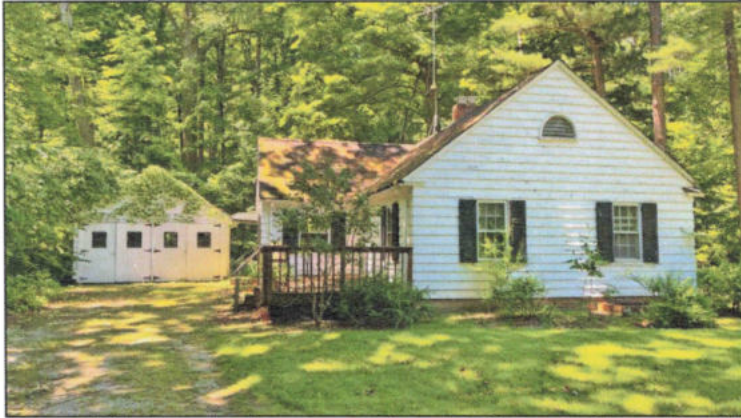
1. Looking west at the western house and garage located in the Building Area in the northeastern corner of the Protected Property.
