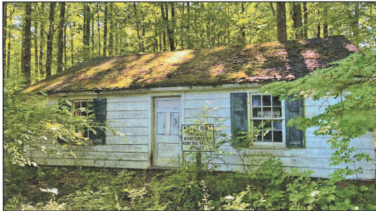
66. Looking west-southwest at the water reservoir building located in the northwestern corner of upland scrub-shrub habitat.
